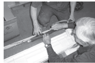
Slice the insulation before bending.
