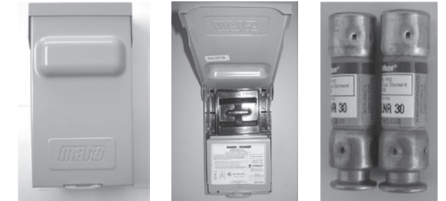
Disconnect switch box for outdoor unit
