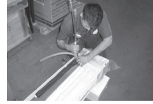
Hold the 90 degree bend root, bend one tube one time, slowly, no quicker than 10 seconds/90 degree bend.
